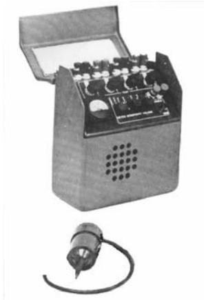
*Texas X150A control unit measuring 7 x 4 x 9 inches shown with one seismometer.*
