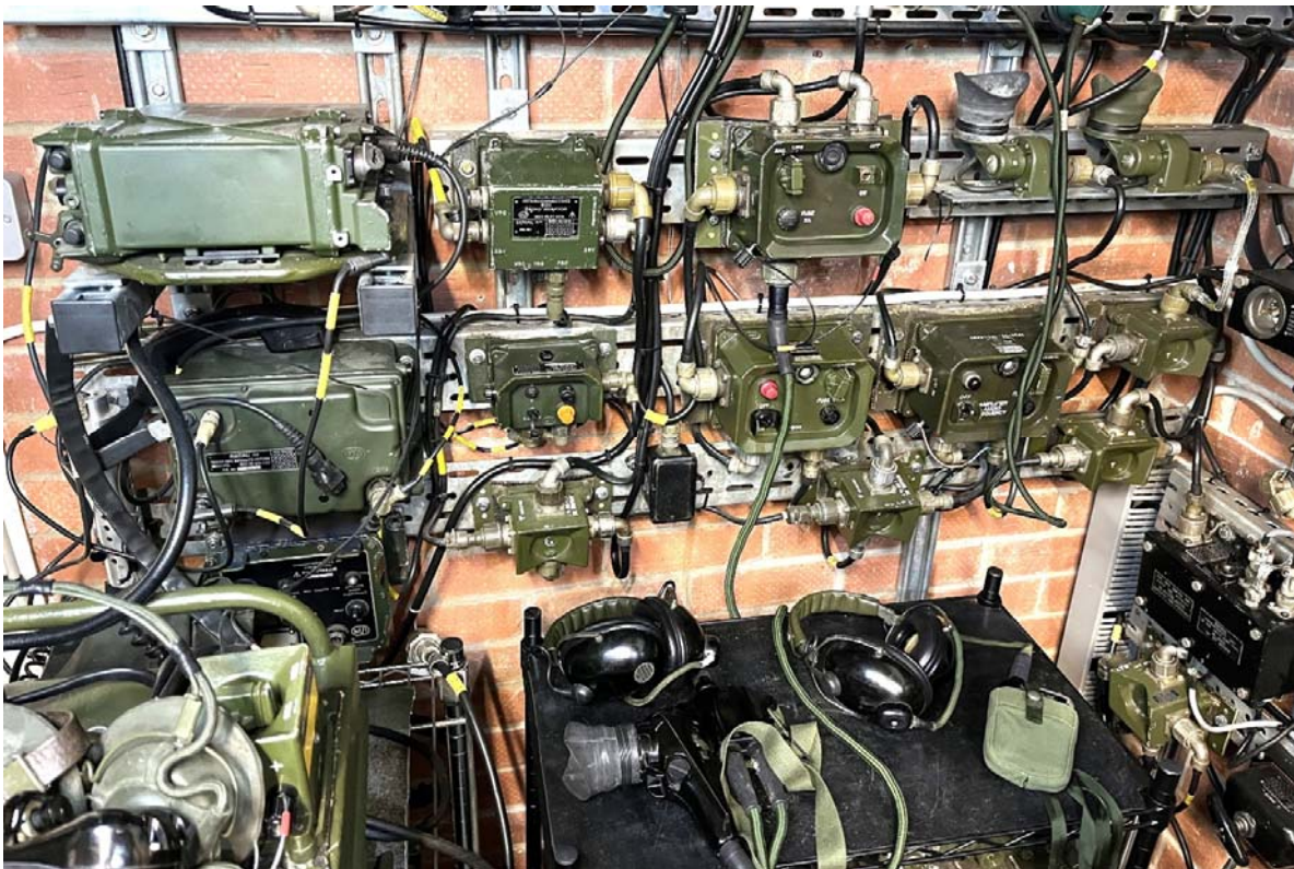
Figure 33. The completed Abbot FV433 installation (excluding the driver's section to the right – see Figure 26). The No. 1's Microphone Magnetic SI No. 9 and the induction loop pocket receiver can be seen at the bottom on the table, complete with the Amplivox E22 noise-reducing headphones. The No. 1's (black) foot acknowledgement switch can be seen on the bottom Dexion rail in the centre
