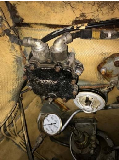
Figure 6. The 'special' induction loop junction box in the turret
